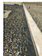
6: Bridging Roof Membrane with Numerous Repairs
