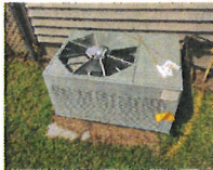
21: Outdated Air Cooled Condensing Unit
