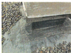
14: Ballasted EPDM Roof with Many Repairs Done
