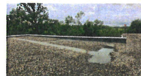
5: Pooling water on Roofs
