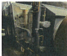
13: Air Handling Unit Well Past Its Useful Life
