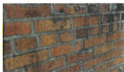
15: Heavily Deteriorated Tuckpointing
